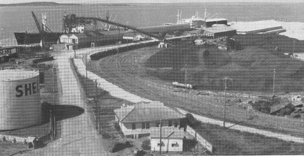
Coal loading facilities, Gladstone
